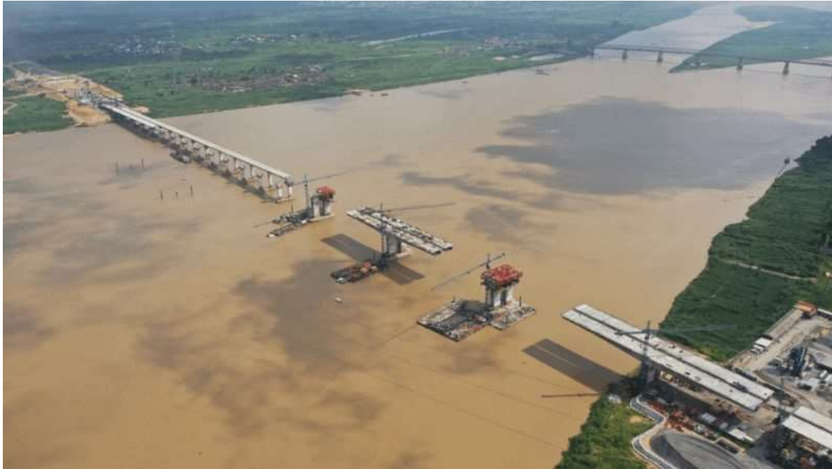
The Second Niger Bridge at Onitsha, Nigeria.
